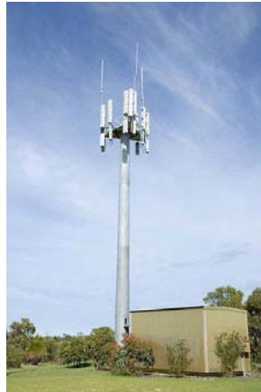
Mobile phone base station
