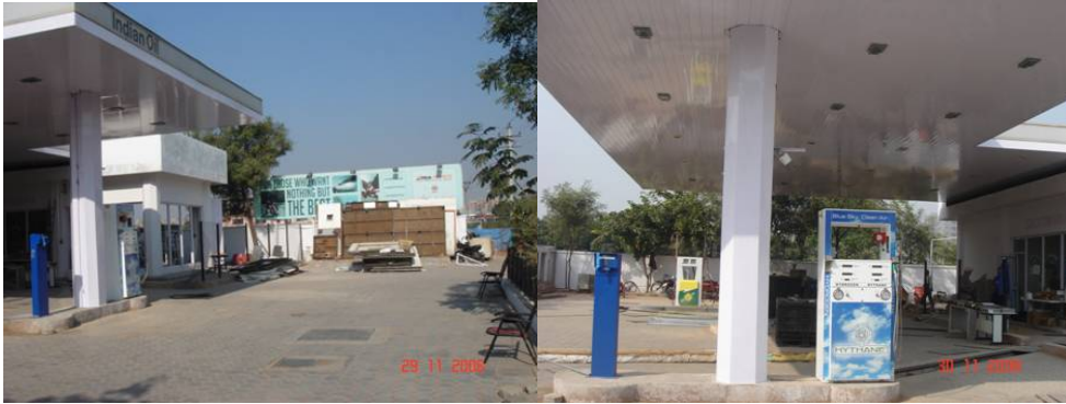
Dwarka Hydrogen-CNG dispensing station (pictures courtesy of Mr D Chenoy (SIAM))
